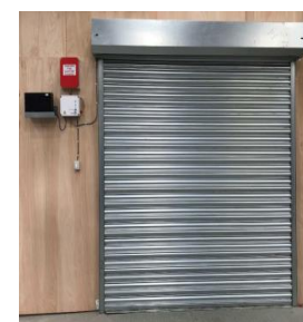
Gravity Fail-Safe Fire Shutter In-house testing without power
